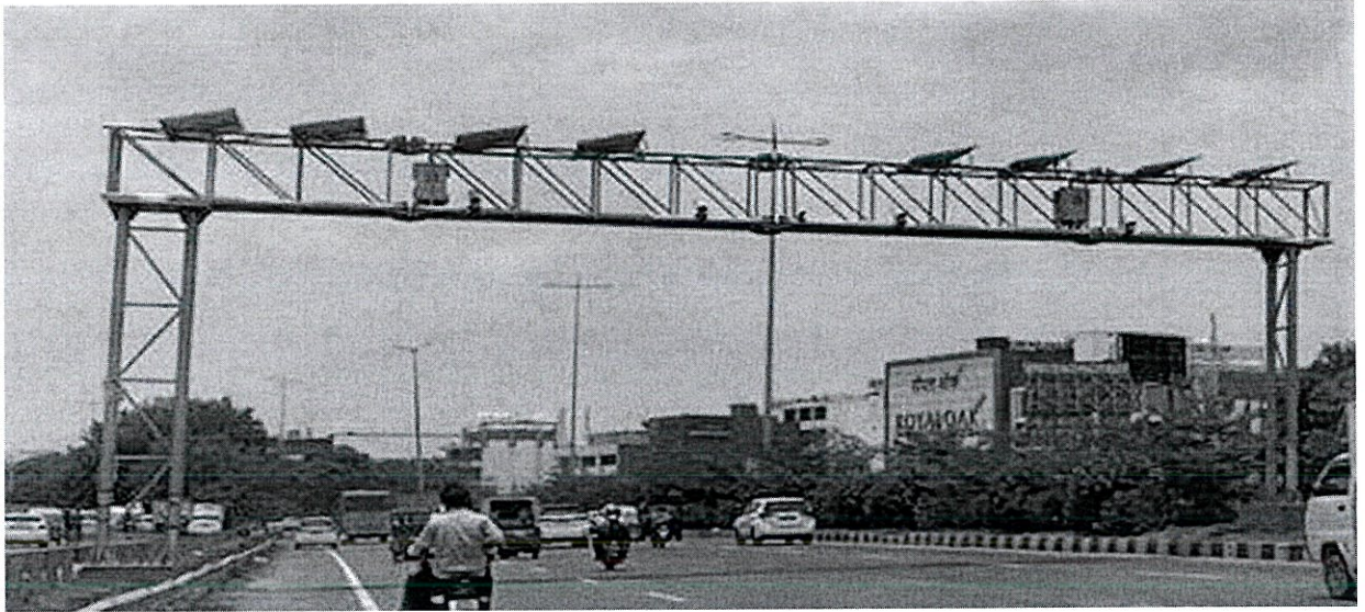
Figure 4: Video Incident Detection & Enforcement System - Dwarka Expressway
