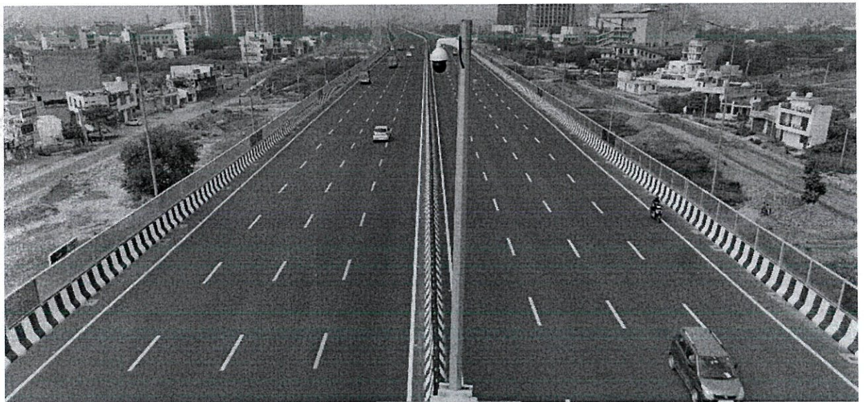
Figure 5: Traffic Monitoring Camera System - Dwarka Expressway
